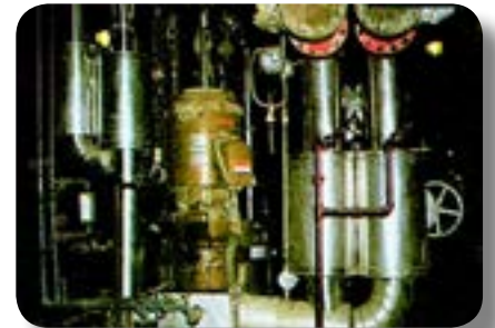
▲ High-temperature LMV-311 installation (temperatures to 650°F)
