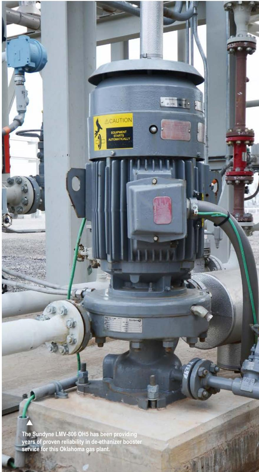
▲ The Sundyne LMV-806 OH5 has been providing years of proven reliability in de-ethanizer booster service for this Oklahoma gas plant.
