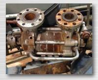
For this university's maintenance team, the set-up caused weekly maintenance work on their segmented-ring pumps. A review of maintenance logs showed that more than 1,600 hours of work was required to keep their ring pumps operating. Thirty-two different work orders were placed
