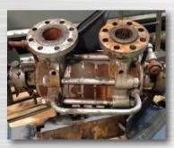
For this university's maintenance team, the set-up caused weekly maintenance work on their segmented-ring pumps. A review of maintenance logs showed that more than 1,600 hours of work was required to keep their ring pumps operating. Thirty-two different work orders were placed
