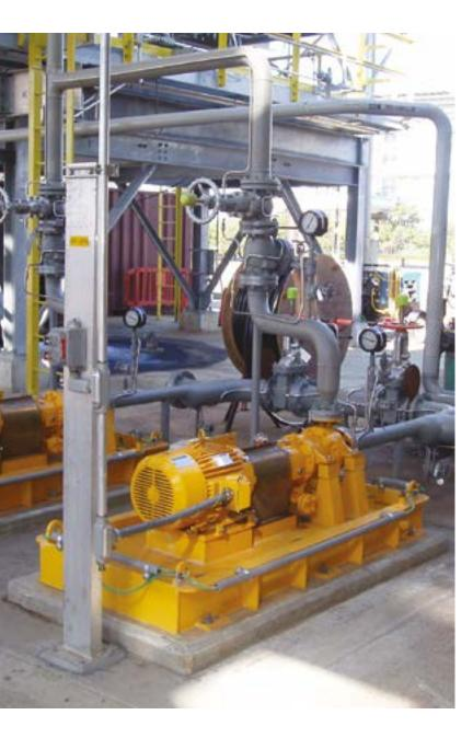
The GSP range comprises of pumps based on the Sundyne HMD Kontro GS drive, built to API 685 specification, suitable for heavy-duty applications.
