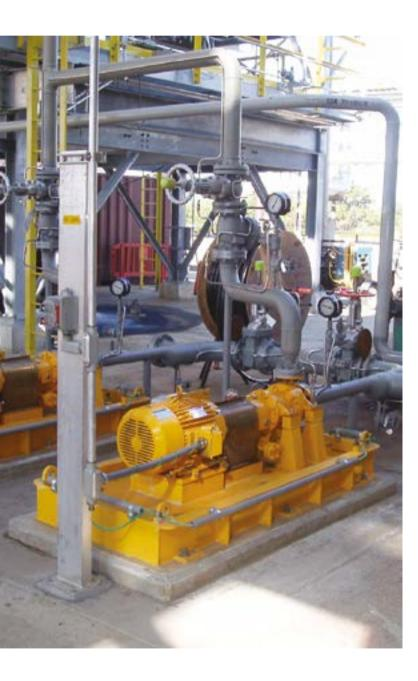
The GSP range comprises of pumps based on the Sundyne HMD Kontro GS drive, built to API 685 specification, suitable for heavy-duty applications.
