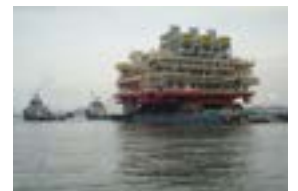
▲ Sundyne centrifugal BMC compressors were installed on this floating production platform in waste gas service off the coast of Abu Dhabi.
