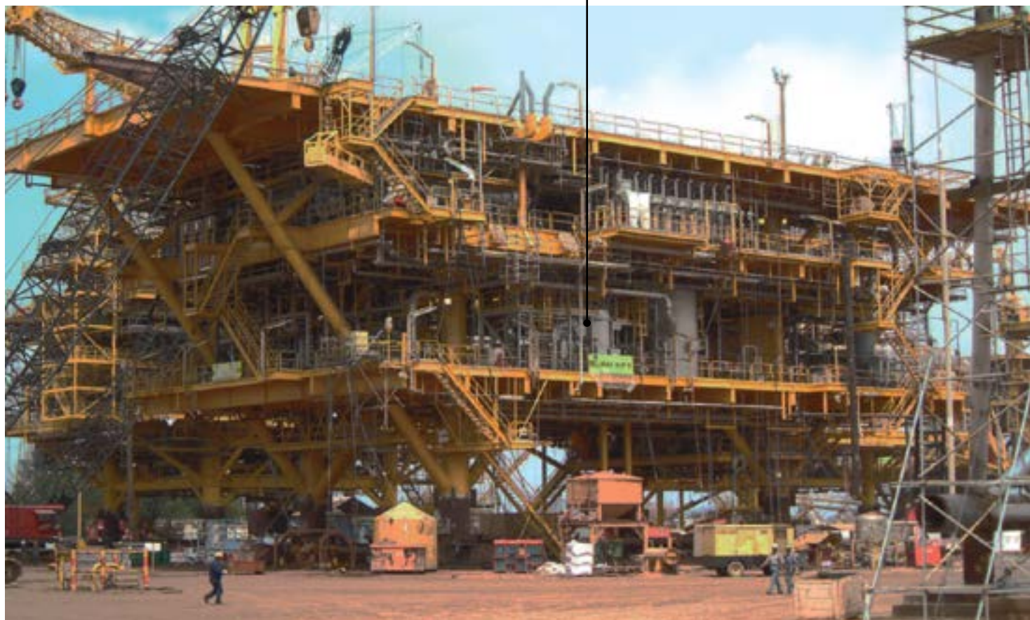
Four Sundyne OH6 pumps installed on two Indonesian production platforms.
